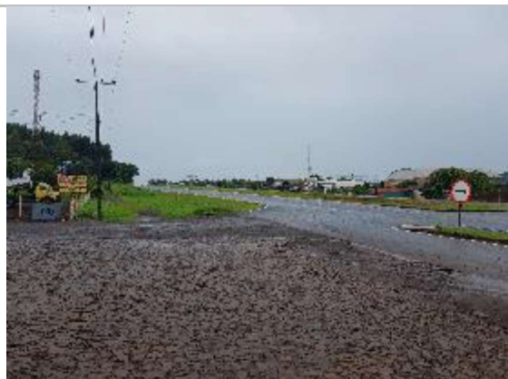
Rodovia BR-277, KM 690
