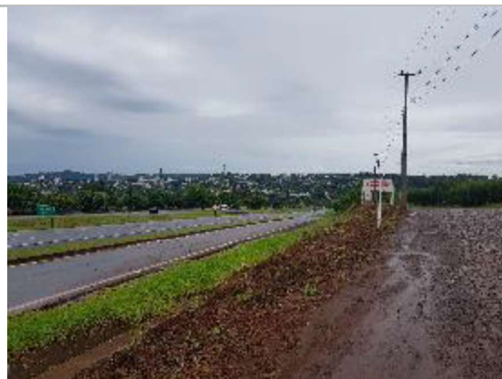
Rodovia BR-277, KM 690
